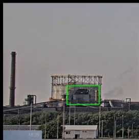
Wrong: No Smoke
